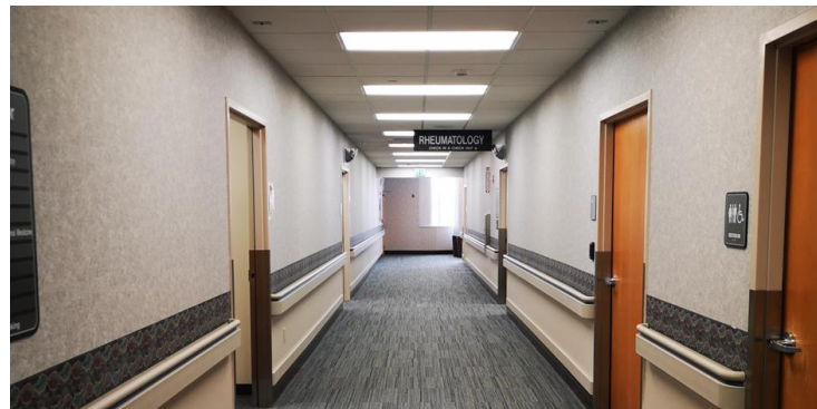
Common Area Flooring Replacement
