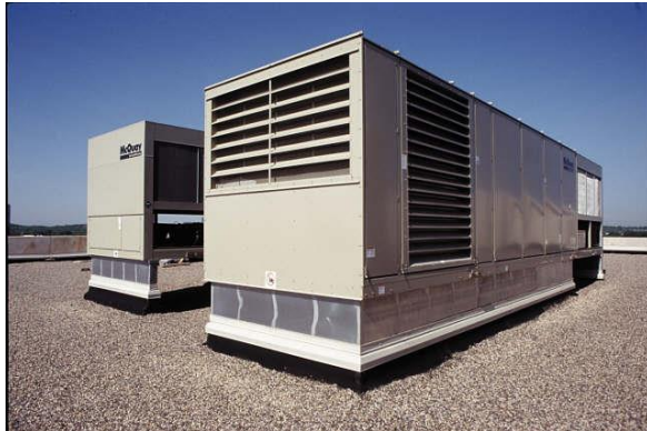
HVAC Unit Replacement
